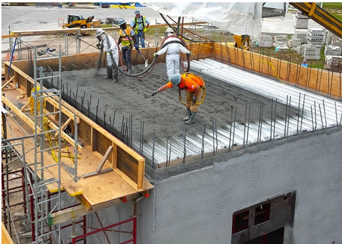
Fig 4: Erection of protected building using EMB3.
